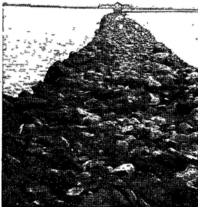
FIGURE 5.—Wall of loko kuapa made of basalt. Weloko Pond, Waimano, Oahu. (B. P. Bishop Museum Negative 3751.)
