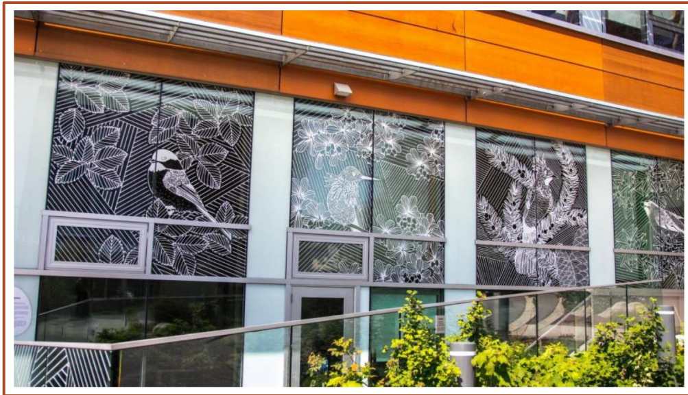
Figure 16: Special applications break the reflection of trees that lures birds into lethal window strikes. In response to a survey showing significant lethal bird collisions with windows on campus (De Groot et al. 2021), the University of British Columbia has developed Bird Friendly Design Guidelines for Buildings as part of a Green Building Plan ( Bird friendly art saves feathered lives (ubc.ca) ).
